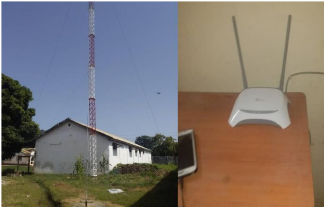
23 Sept 2020, cell tower and internet connection at Mile 2
